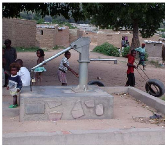
Fig 1. Typical abandoned handpump , abandoned within 3 years due to missing spare parts.
